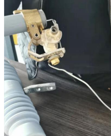
8. Cut off the excess fuse link
