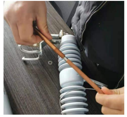
5. Screw the fuse link into the cap
