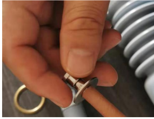
1. Loosen the nut of the fuse
